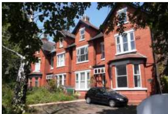
Residential properties along Regent Road. Some have replaced traditional timber windows with uPVC and faux-leaded lights
