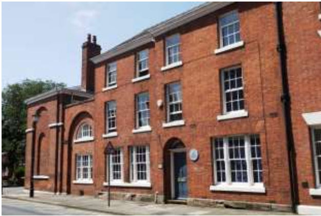
Late 18 th century buildings along Market Street
