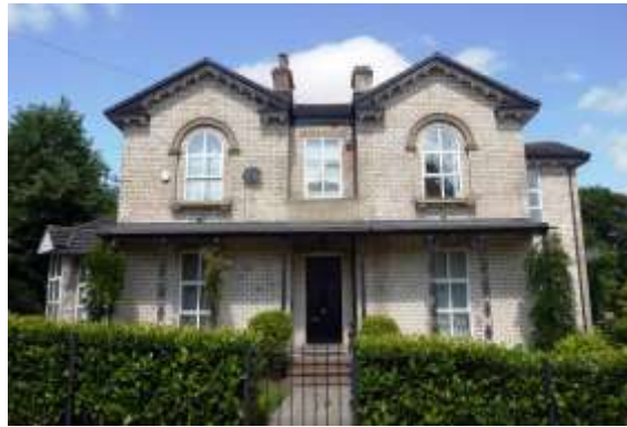
Example of the typical architectural features of the area including deep eaves and brackets and wide buff bricks. Windows have been replaced with inappropriate uPVC windows and an unsightly extension has been added (left of image)
