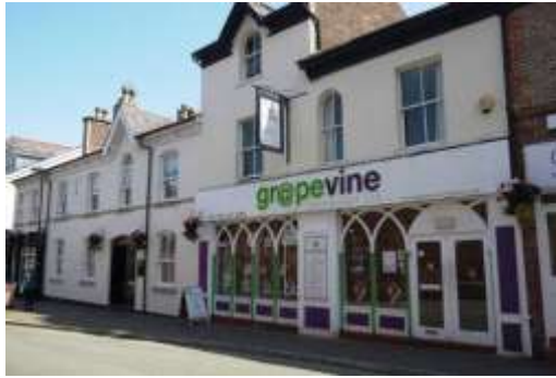
Traditional 'Gothic' window frames are harmed by an intrusive colour scheme and modern signage
