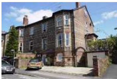
Raised gardens have been removed from Springfield Road to create additional living space, often without sensitivity to the historic surroundings and using uPVC windows
