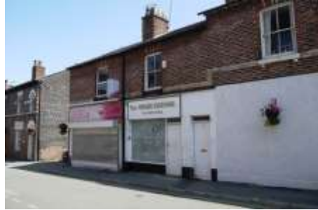
Vacant shops along Greenwood Street with inappropriate security features, render and signage
