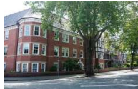
Modern development on Groby Road that takes design cues from the surrounding Arts and Crafts architecture but is rather monumental in scale
