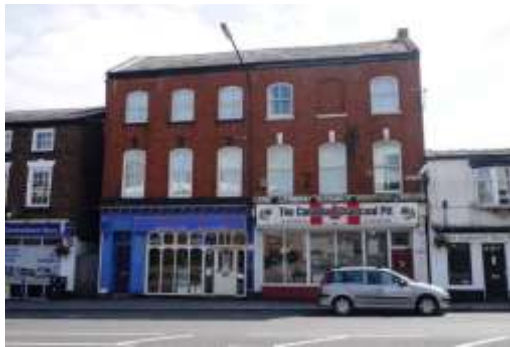
Inappropriate signage and colour schemes dominate traditional features that do survive such as brackets and fanlights
