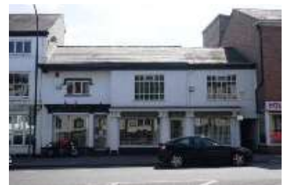
Good example of traditional shop fronts at 14-18 Old Market Place (but replacement glazing and doors and painted brickwork)
