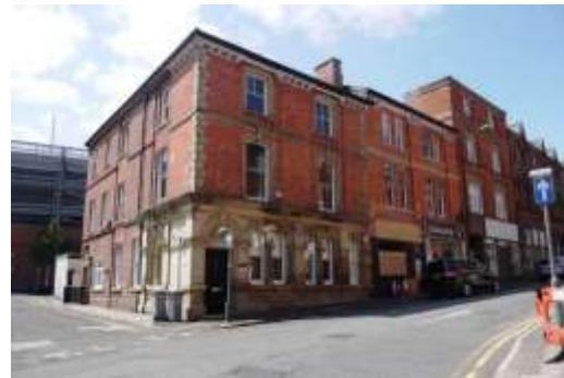
Buildings on the corner of Stamford Street and Kingsway in a good condition but with recently vacant shop units
