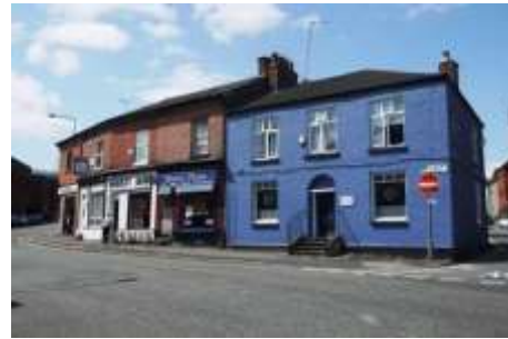
Inappropriate painted brickwork on Stamford Street
