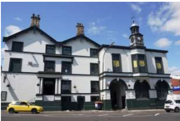
Old Market Tavern incorporating the old Town Hall
