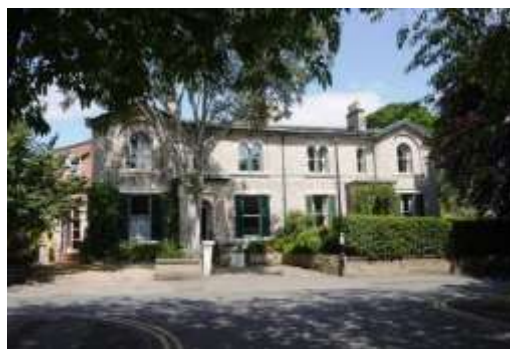
2-4 The Mount, well maintained but some loss of boundary treatments to create parking
