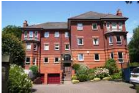
Modern detached development within the residential areas
