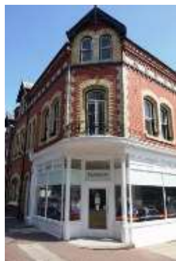
Example of a good shop front on Market Street
