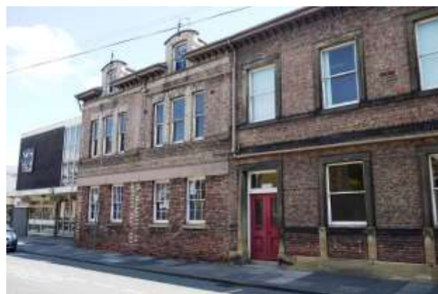
Various phases of development seen across the Altrincham Hospital site
