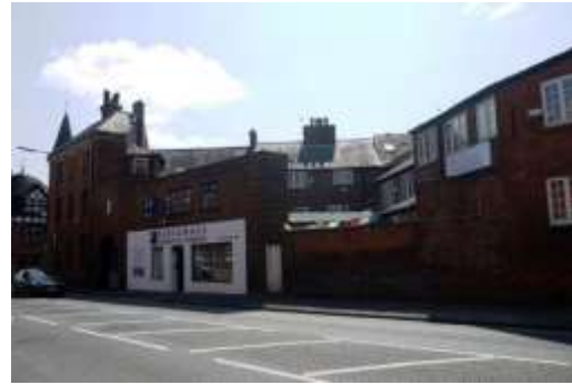
Inappropriate modern shop front jarring with the historic surroundings
