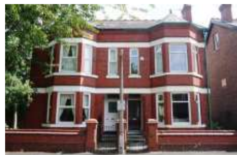
Example of the residential properties on Richmond Road with distinctive white painted banding. Window replacement is a common concern in this area but boundary walls have been retained to all properties.
