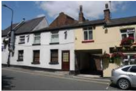
Replacement windows and doors are detrimental to these late 18 th century properties, particularly the faux-leaded lights
