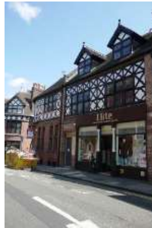
Example of an appropriate shop front
