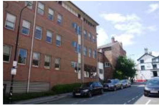
Modern development that is out of scale with the historic core of the Conservation Area, particularly the characteristic variation in heights seen between each property along most streets
