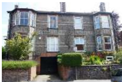
Some properties along Springfield Road retain their raised gardens but garaging has been inserted at basement level
