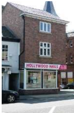
Inappropriate signage within the historic core of the Conservation Area
