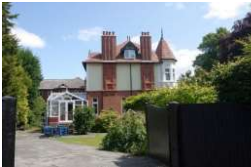
Doonfoot House, Regent Road is a high-quality residential property in a good condition. The modern conservatory somewhat detracts from the Conservation Area.
