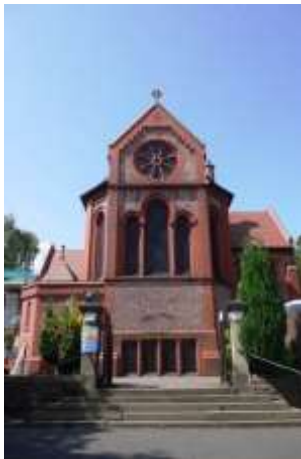
East end of Church of St George
